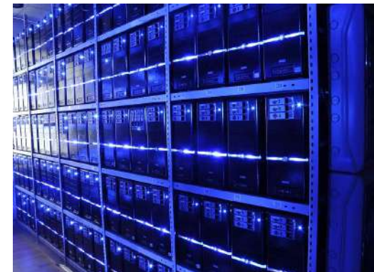
EMR Site, Bidder Street, E16 4ST
