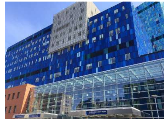
Whitechapel Road development site, E1 2BB
